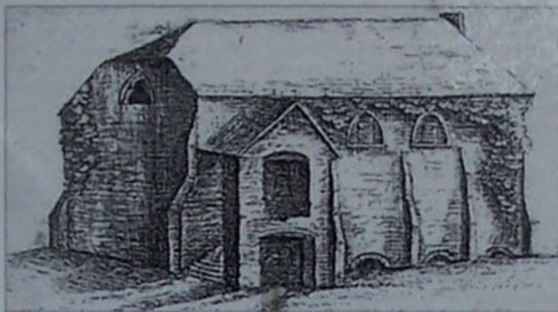
(Above) A water-colour drawing made by John B Swete in 1780. The half-hipped roof at the western end is likely to be a post-medieval alteration. The windows appear to have been partially blocked up; note the tracery shown in the head of the west window.
